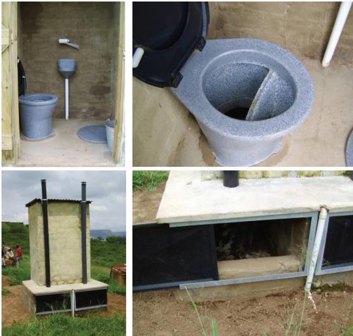
**Figure S2.** A UD-VIV latrine – top left: front view showing the urine-diverting pedestal seat unit, urinal, and cover over the entrance to the vault not in use; top right: close-up of the urine-diverting pedestal seat unit; bottom left: rear view showing the two vent pipes (one for each vault) and the small urine pipe (in the centre) which leads to an adjacent soakaway; and bottom right: close-up of one of the two vaults with the sliding door open showing the dehydrating vault contents.
